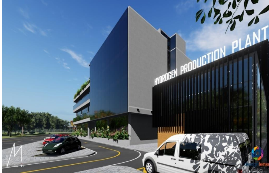
Hydrogen production plant (under construction)
