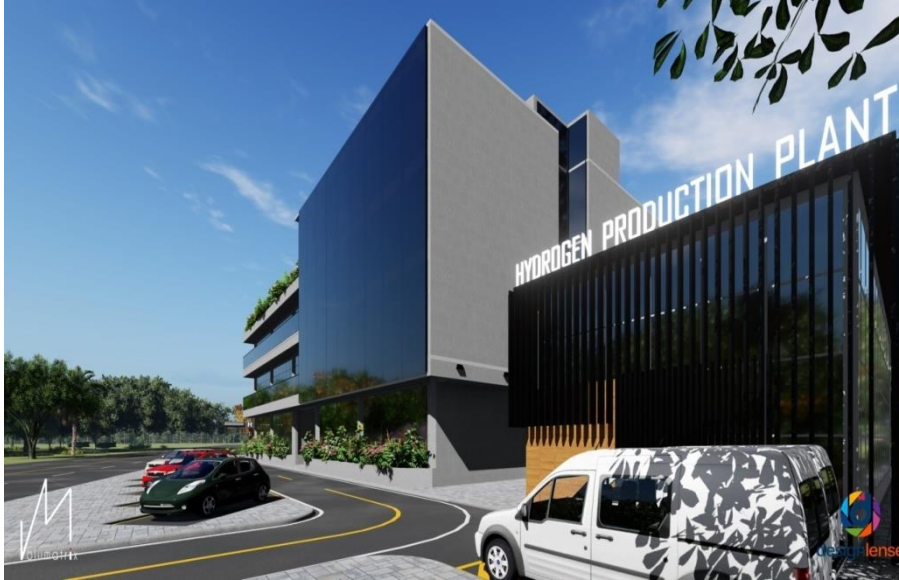
Hydrogen production plant (under construction)
